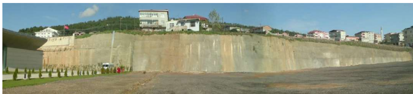
Figure 7. General View of Soil Nailing Area.
